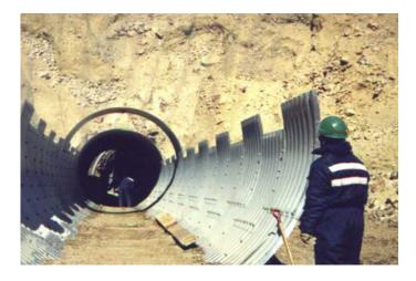
TV 100 corrugation makes this solution the most efficient alternative for structures with diameter between 1.8 and 3.8 meters. Compared to tunnel installations, TV 100 Multi-plate requires a lower height of the soil over the top between the structure keystone and the soil level, which implies that this is an ideal solution for superficial installation. Nevertheless, its structural robustness allows it to be installed in very deep places.
